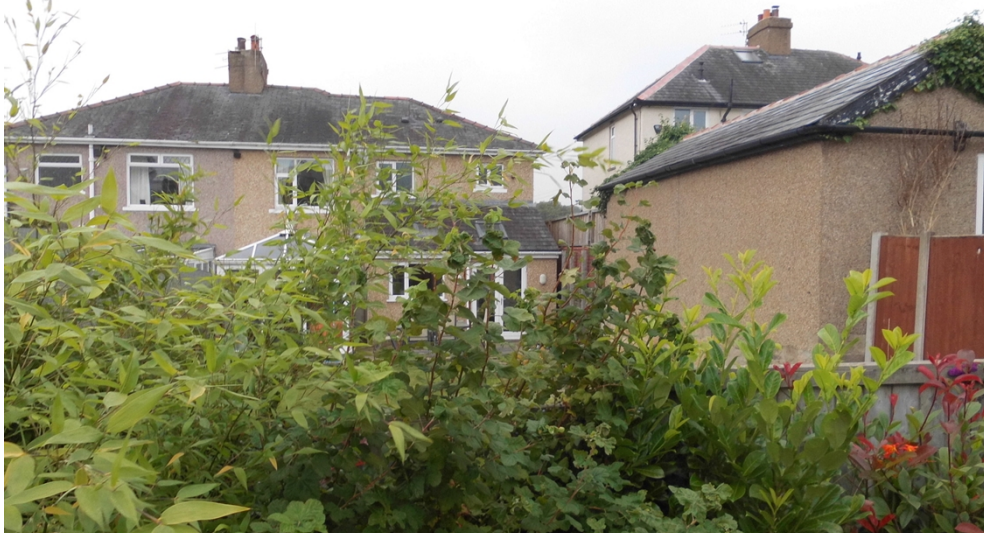
rear boundary fence / rear of houses on Slade Lane Page 79
