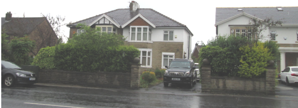
Existing pair of semi-detached houses
